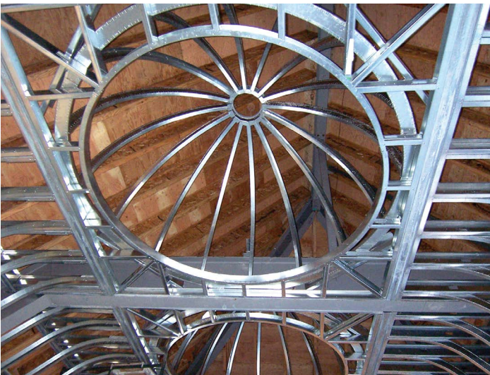
Interior Ceiling Domes
