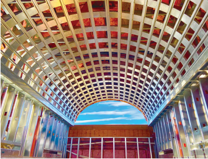
Arched Tracked Barrel Ceiling
