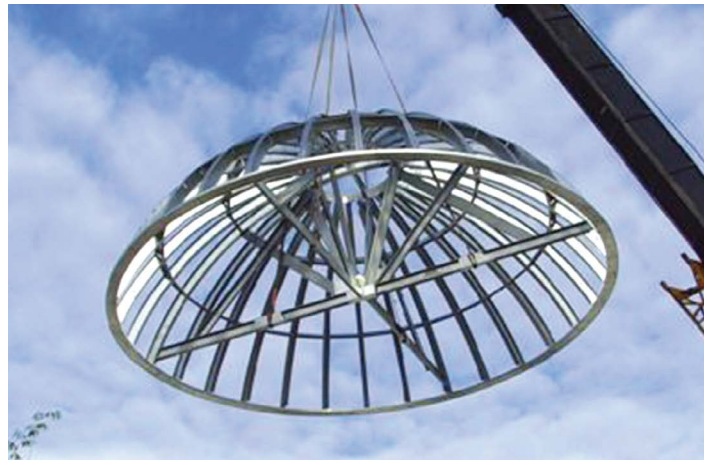
Exterior Roof Domes
