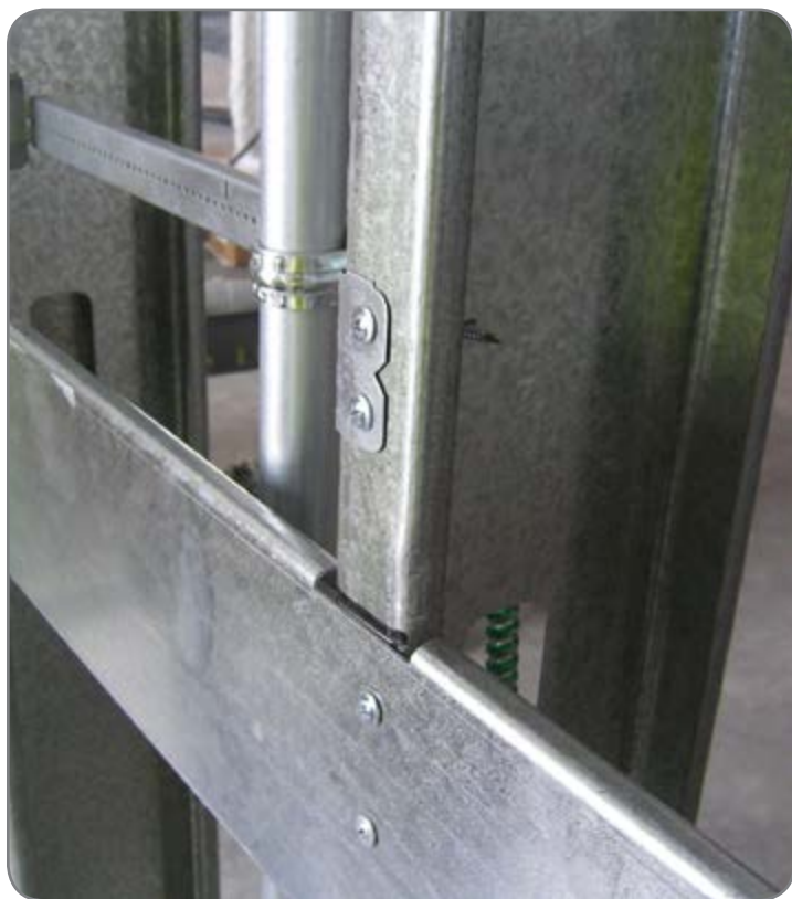
Image of Notched Stud Backing, demonstrating attachment to stud.
