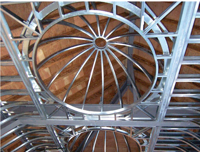
Interior Ceiling Domes
