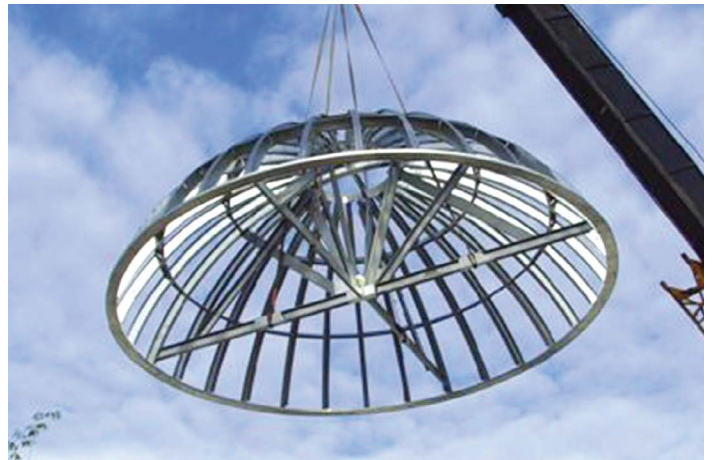
Exterior Roof Domes
